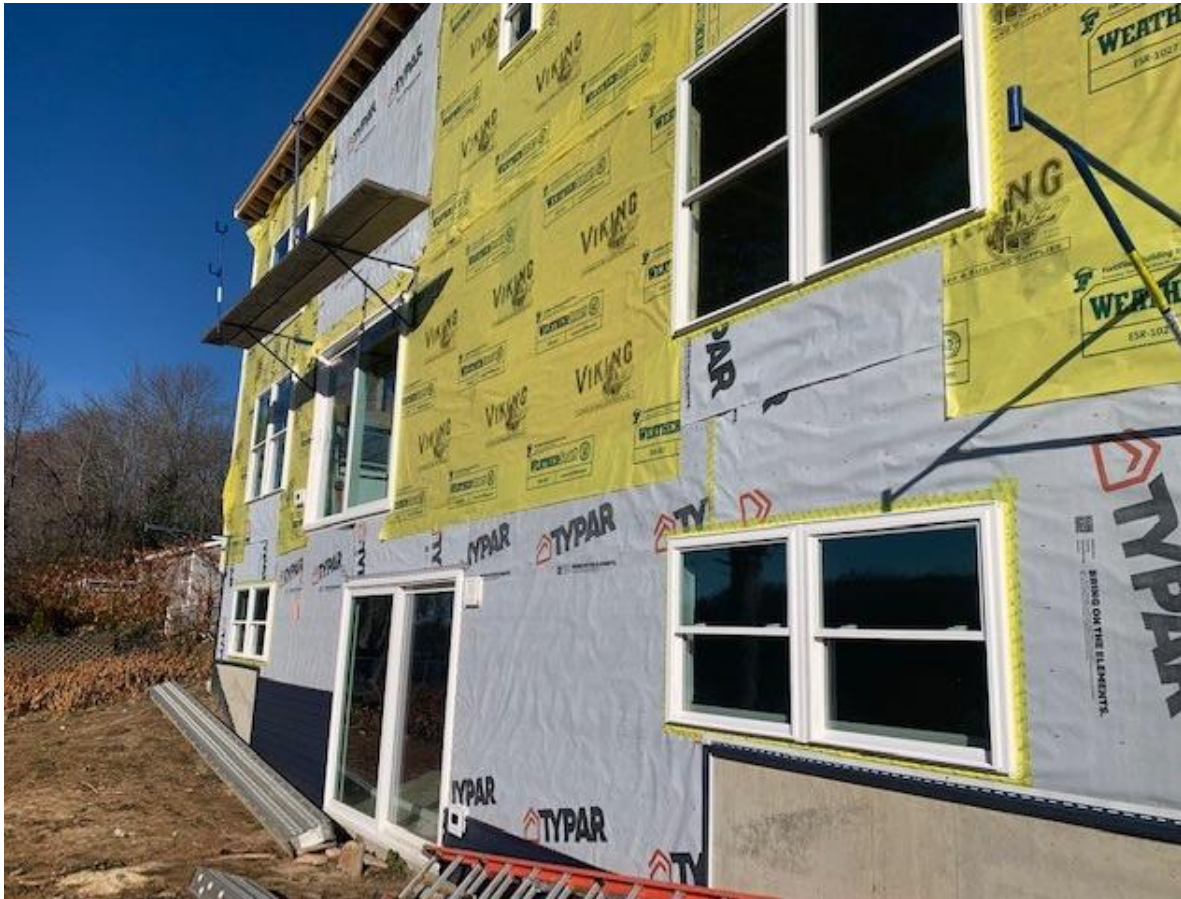
New Home Construction taking place on Indian Island, Maine
