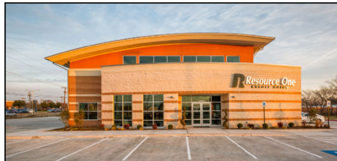
Resource One Credit Union branch in Garland, TX.
